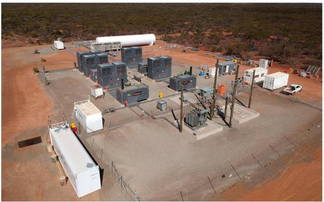
Figure 4: New Power Station with LNG facility in background pre-commissioned
